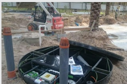
► Treatment plant during installation.
