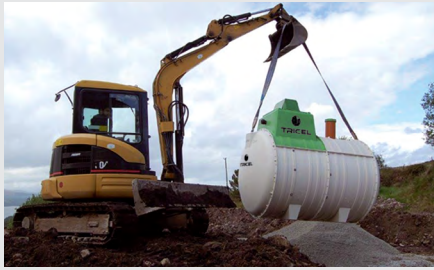
▶ Tricel Vitae 6 being installed
