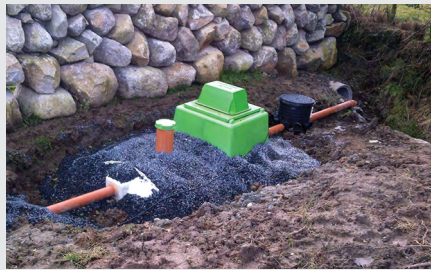
▶ Tricel Vitae 6 installed
