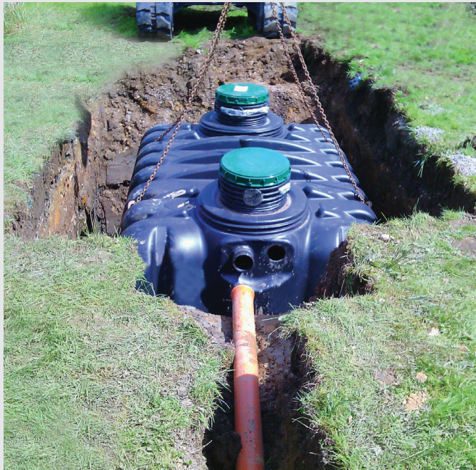
Tricel Vento installed.
